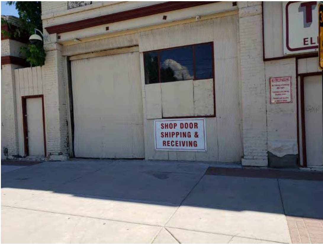
Existing drive entry for Thomas Electric
