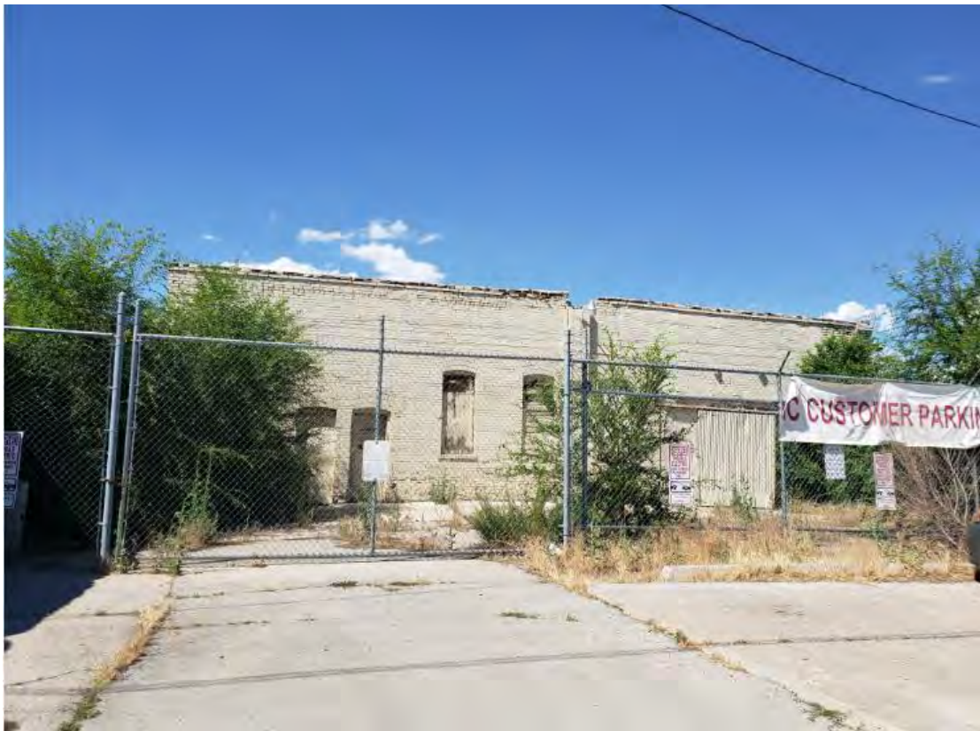
Rear of existing building
