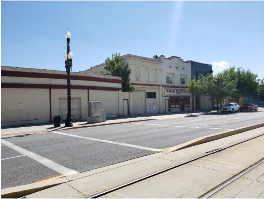
Site (Thomas Electric – tan buildings – to be removed)
